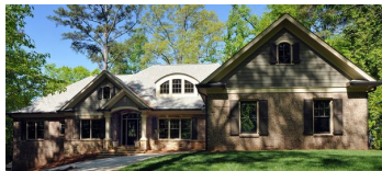
A 5,500-square-foot custom home in Brookhaven was designed by Healthy House of Georgia with character and a focus on air quality, and water and energy efficiency. Photo Credit: Dennis McConnell
